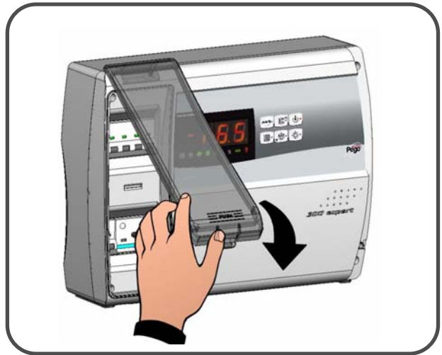
Fig. 4: Close the transparent protection cover.
